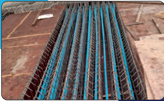
Installation of Unbonded PT System
