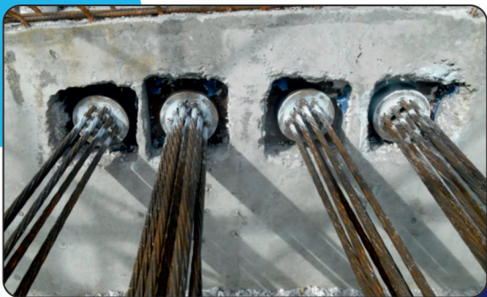
After concreting of Bonded PT System
