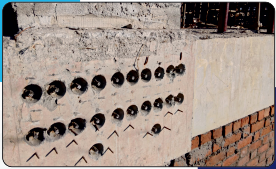
Beam After PT Cable Cutting
