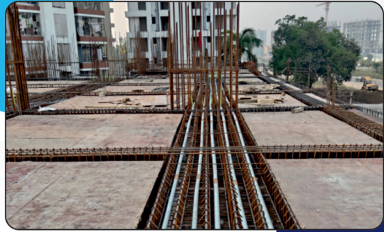
Installation of Bonded PT System
