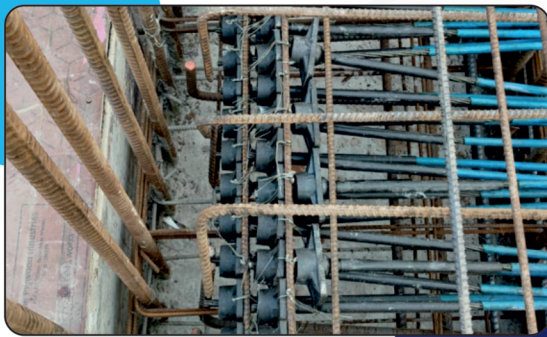
Dead End of Unbonded PT System
